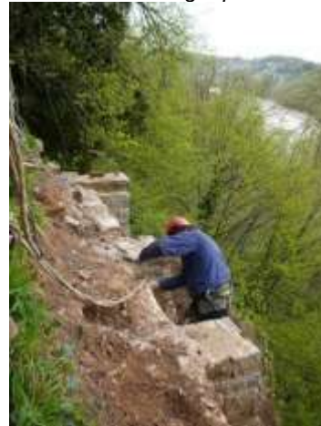
Repair of buttresses using roped access (2009)
