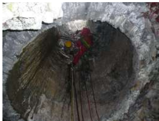
Interior pining of main furnace flue
